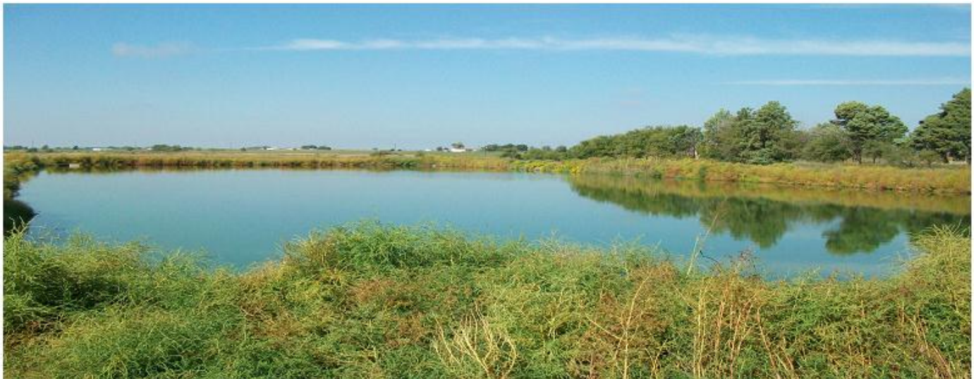
Figure-4. Oxidation pond treatment system.
